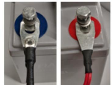
Use the supplied cable with U spade terminals directly for battery/cell wiring
